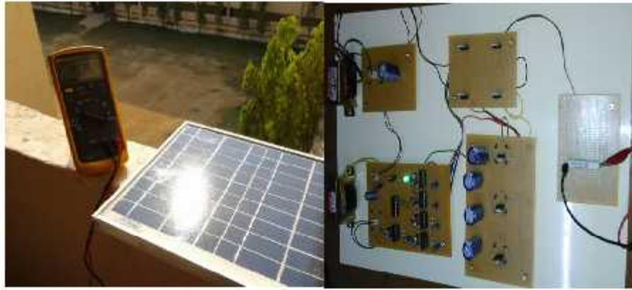
Fig.13. Setup of the 1211-SUNSTAR solar panel and multi-level inverter
